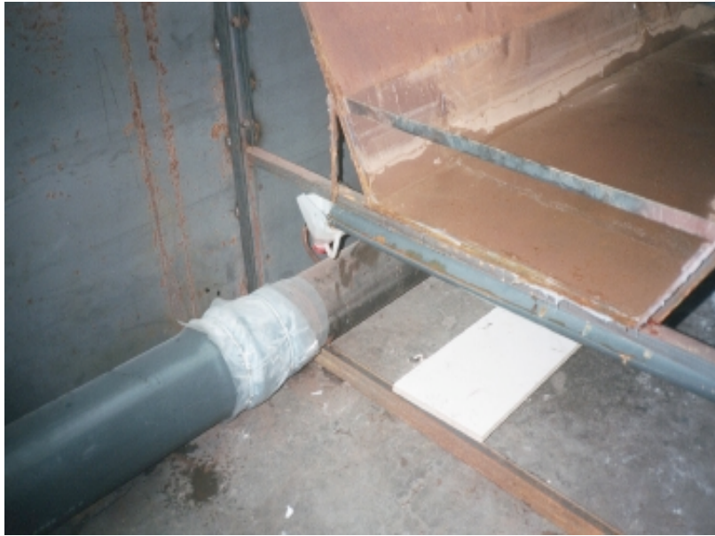
Fig. 6: Detail of channel components I und II (left site): Provisional sealing of the tube and gutter for dripping water (1993) (photo:: Jochen Saueracker)
