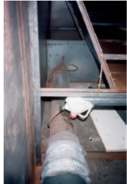
Fig. 7: The dripping water was led through a thin hose to the basin. (1993) (photo:: Jochen Saueracker)
