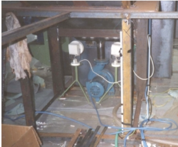
Fig. 4: View of the original lighting: white spotlights with green painted tripods (1993) (photo: Jochen Saueracker)
