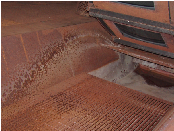
Fig. 6: Channel component V, splash water area beneath the wheel after ten months of presentation: compared to fig. 3 the development of corrosion become apparent (August 2005) (photo: ZKM)
