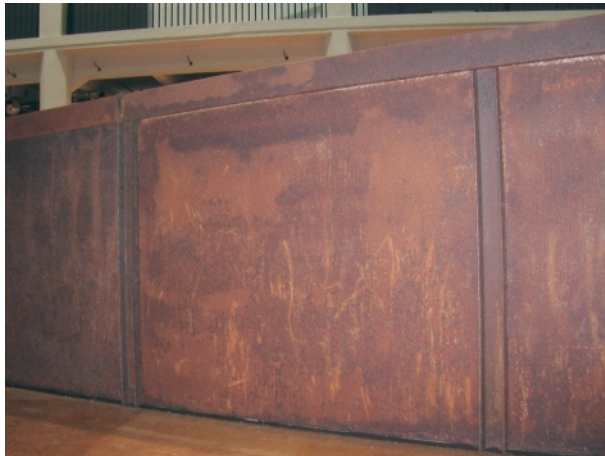
Fig. 1: Channel component III showing damage by abrasion of rust surface (bright red wipe traces) (March 2006) (photo: ZKM)
