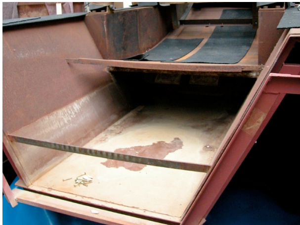
Fig. 3: Detail of water channel component V showing old calcium carbonate deposits from 1993 (August 2004) (photo: ZKM)
