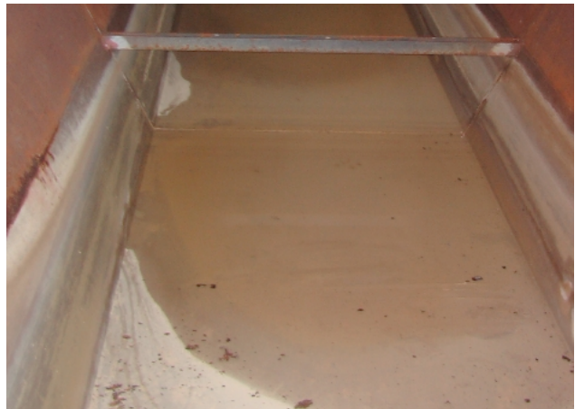
Fig. 4: Detail of the water channel with a strong layer of calcium carbonate after two years presentation (October 2006) (photo: ZKM)
