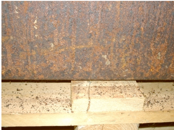
Fig. 2: Detail of the channel's outside with lightly adhering encrusted areas and loose rust particles (September 2004) (photo: ZKM)
