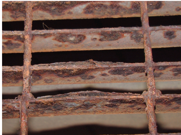
Fig. 11: Detail of the grille: detached corrosion layers (March 2006) (photo: ZKM)
