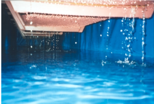
Fig. 5: Space underneath the tank panels: during operation water runs through the joints between the tank panels (photo: ZKM)
