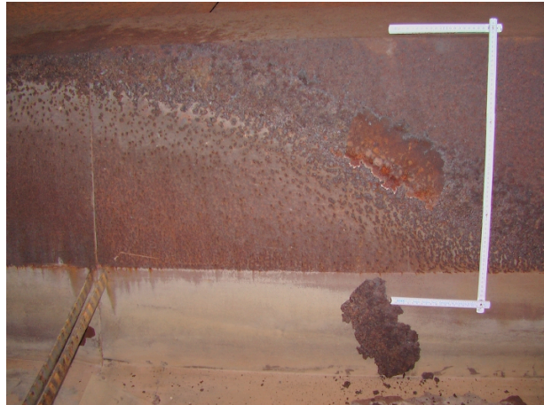
Fig. 9: Detail of splash water area, right side of water tank: Partial loss of corrosion layer (March 2006) (photo: ZKM)
