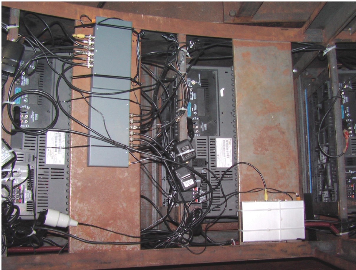
Fig. 16: View of one of the wheel segments where the new flash card player (silver) and two of the new video distributors (grey) are fixed during testing phase. (May 2005) (photo: ZKM)
