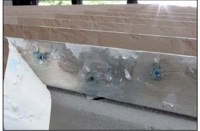
During Treatment: Detail showing the blue corrosio at the copper rivet interface
