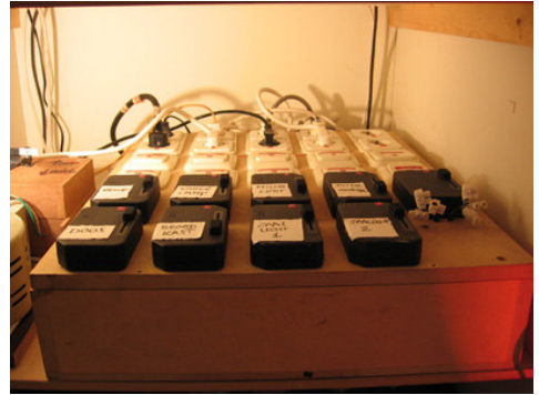
12. Dimmers in the control box
