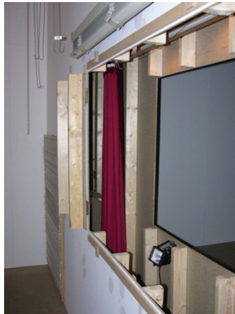
1. The window with the red curtains
