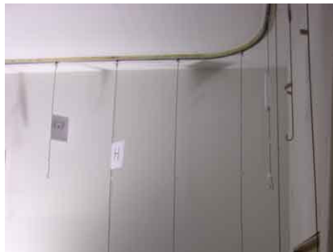
1. The steel rods on the rail
