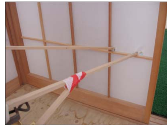
Two slats are nailed to one of the panels to support the construction.
