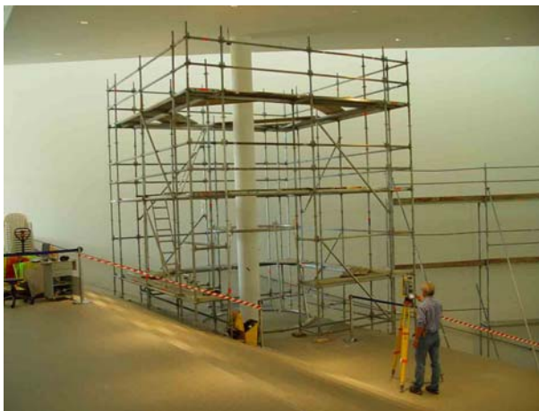
Fig. 46: Tachymetric measurement of the measuring points on the colour lengths.
