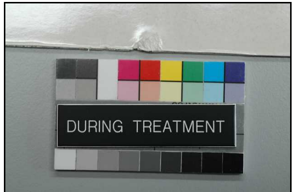
During treatment: detail showing gauge after flattening
