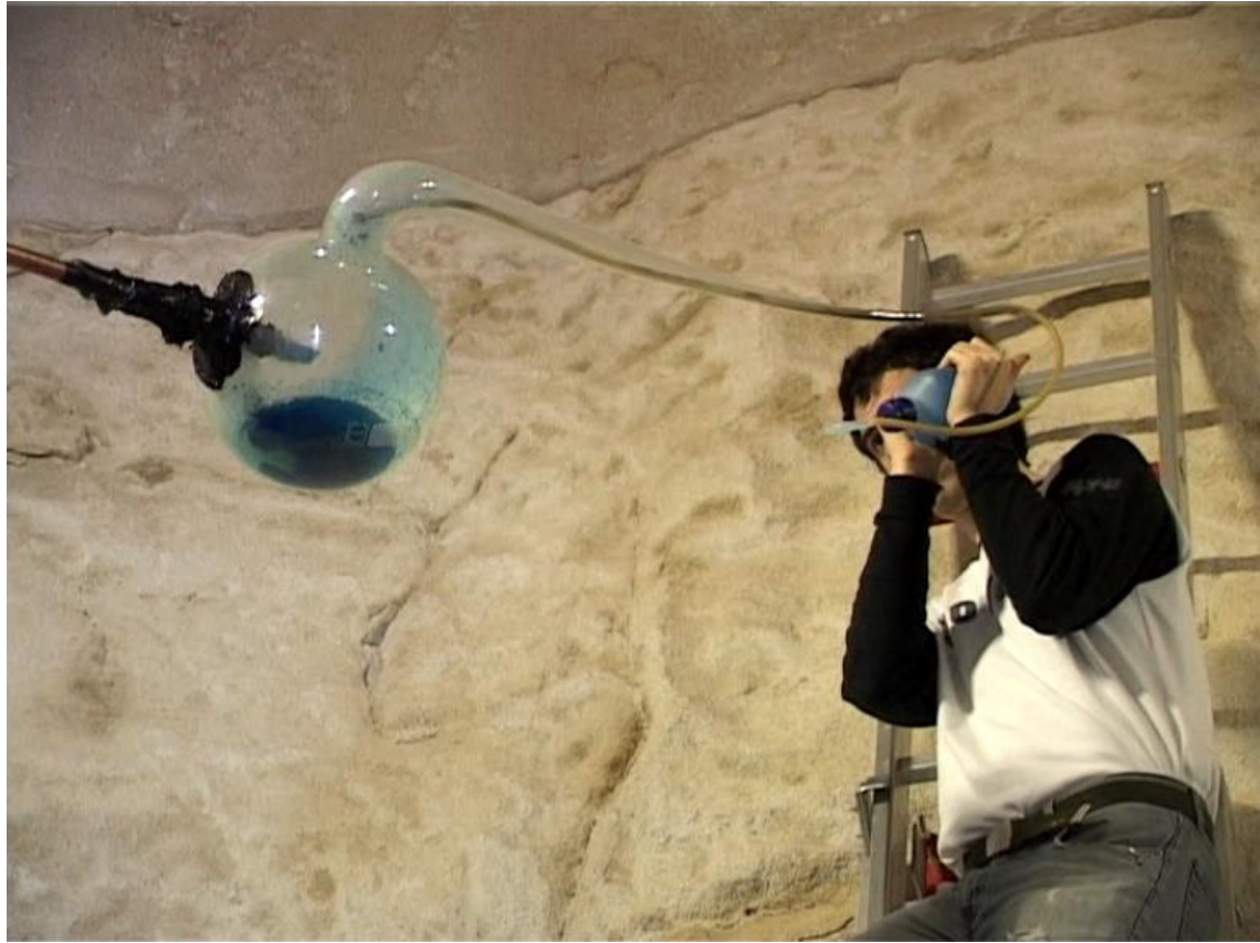
Moment of introducing the copper sulphate dissolved in water with the aid of a plastic I.V. drip.
