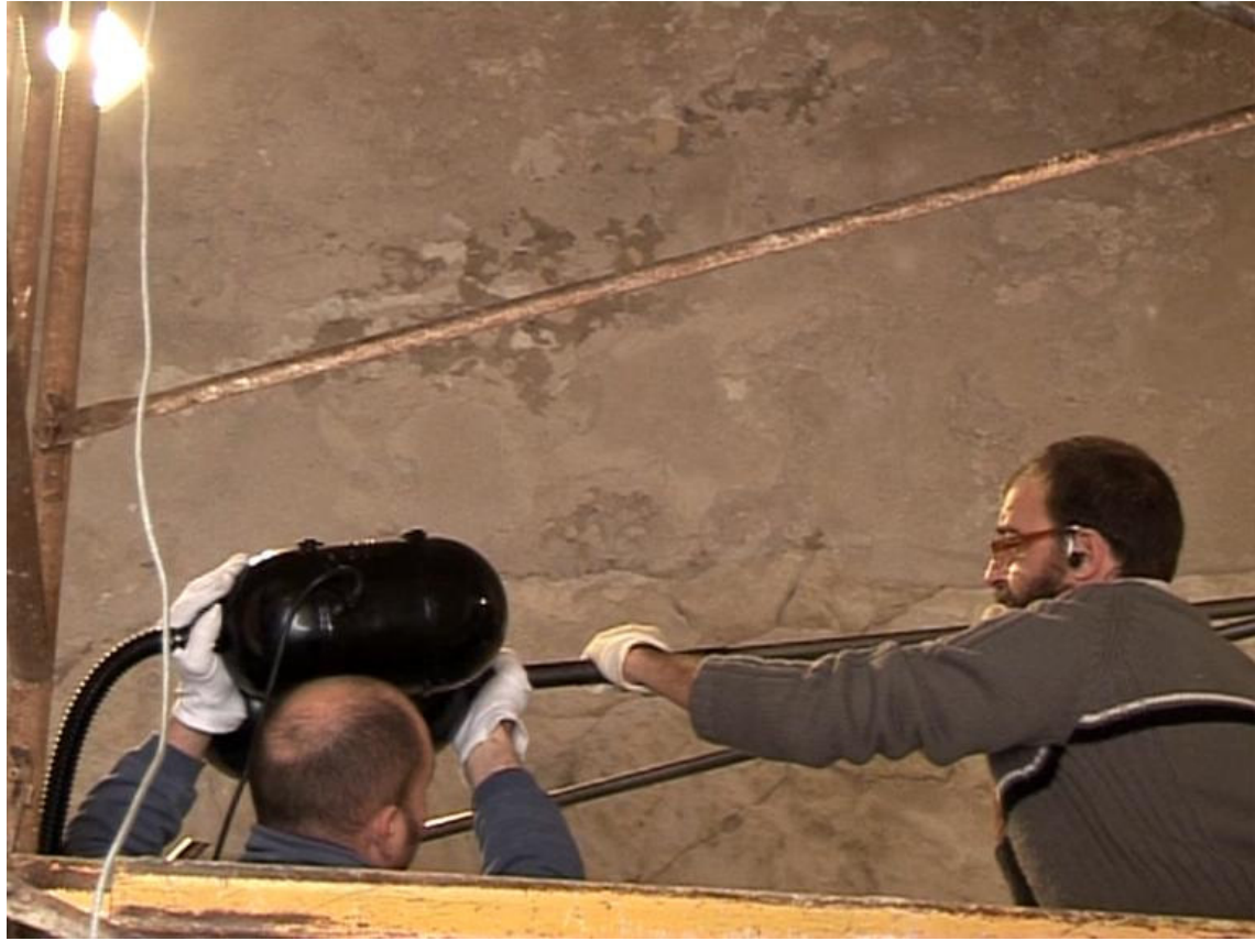
Putting the compressor in place.
