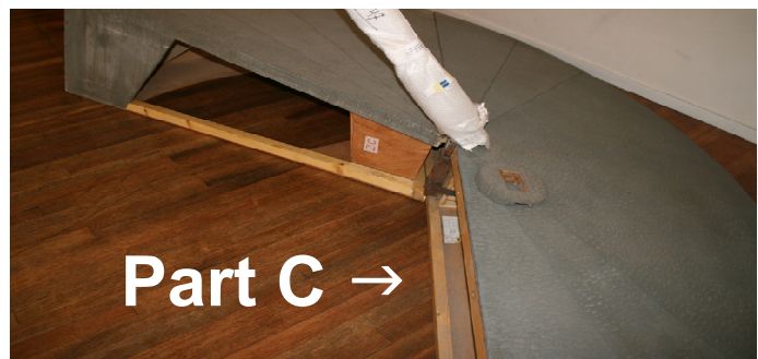
3. Segment A, B and C are assembled with 14 M10 bolts and nuts. Part A and B are connected with bolts 1 to 7 (see construction drawing on next page), bolt 1 is placed in opposite direction (nut facing front). The bolts to connect segment C are placed similarly, but mirrored!
